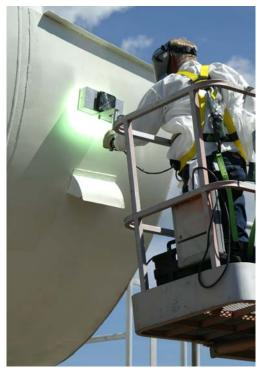
Figure 2. Field Application And Cure Of UV Technology At Warm Temperatures
