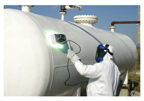
Figure 1. Field Application And Cure Of UV Technology At Cold Temperatures
